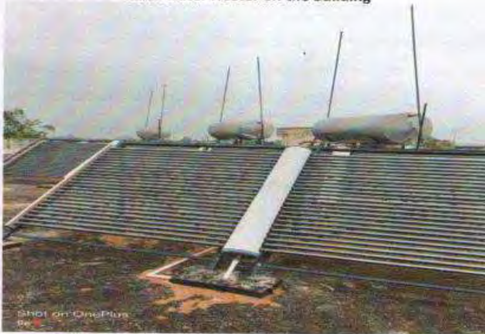
Solar water Heater on the Building
