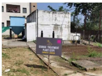
Sewerage Treatment Plant
